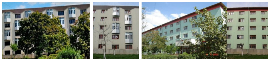
Fig. 2 – Thermally rehabilitated student dormitories in the Tudor Vladimirescu campus: the T14 building covered with POLYALPAN strips, triple glazing and bow-windows for greenhouse effect; the T15 building covered with OLTPAN strips.
