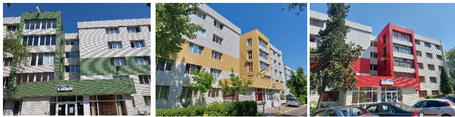
Fig. 3 – Thermally rehabilitated student dormitories in the Tudor Vladimirescu campus: the T9, T10 and T11 buildings rehabilitated at the level of the facades using ventilated façade system.
