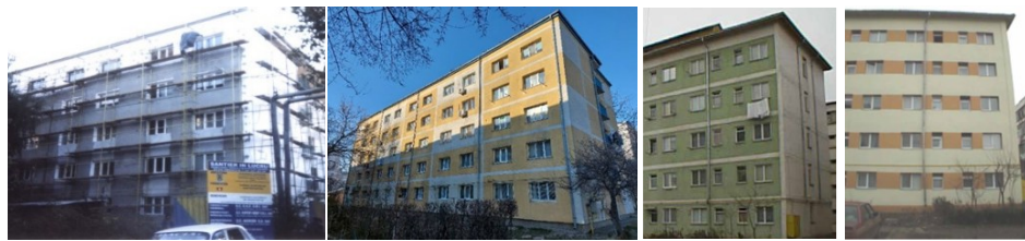
Fig. 1 – The blocks in Iași, Tabacului street and in Piatra Neamț, Progresului street, before and after the execution of thermal rehabilitation works.
