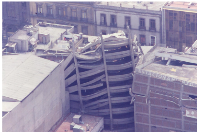
Fig. 9 – “Collapse of precast concrete parking structure due to pounding against adjacent structure in Mexico City (1985 Michoacan Earthquake)” (FIB 27, 2003).
