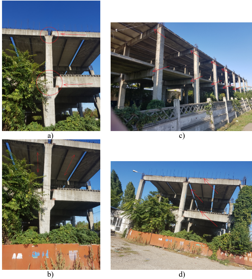
Fig. 10 – The representation of: (a) PRC beams with pin configuration in marginal areas (without any monolithic concrete); (b) the one-way pin supported mode of PHC slab strips on existing PRC beams; (c) prefabricated RC beams on a single global direction of the structural system (along the span direction); (d) the non-existence of an additional top layer of concrete on the PHC slab strips.
