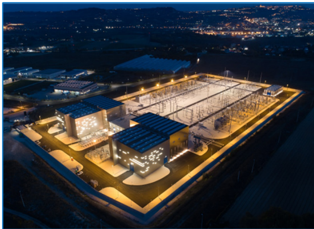
Figure 4: An existing HVDC Converter Station characterized by its exclusive architectural design
