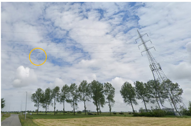
Figure 6: Two parallel spans next to each other equipped with Ampacimon sensors, both installed on the lowest phase (view from maps.google.com)
