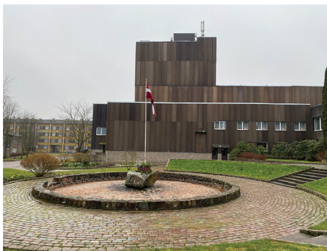
Fig. 8. Kalni Culture House, Saldus district. Architect Ausma Īvāne, 1987. Photo by A. Uškāns, 2025.
