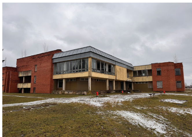
Fig. 2. Abandoned administrative-cultural centre in Rundāni, Ludza district. Architect Laimonis Tīkmanis, 1982–1987. Photo by A. Uškāns, 2024.
