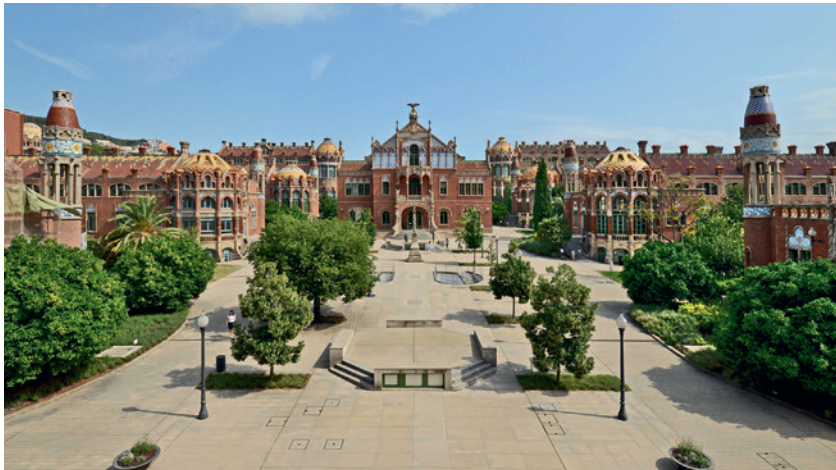
Fig. 31. Hospital de Sant Pau. View from the administration building.
