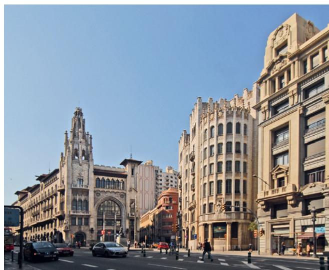
Fig. 49. Caixa de Pensions, Via Laietana, 56-58, (1914–1917), left, and office building Casal de la Previsió, Jonqueres, 2 (1920, in the middle. Enric Sagnier i Villavecchia.
