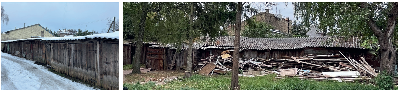
Fig. 9. Storage shed or woodshed.
