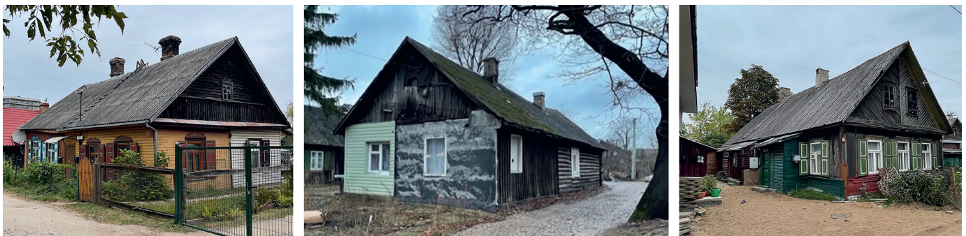
Fig. 7. "Patched-up" buildings [photos by the author].
