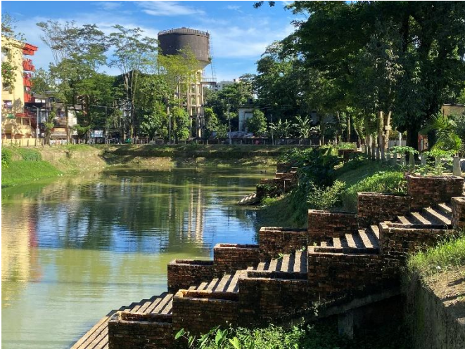
Fig. 22. Pond deck development for public use and recreation at Dostidar Dighi. (Photo: Authors, 2024)
