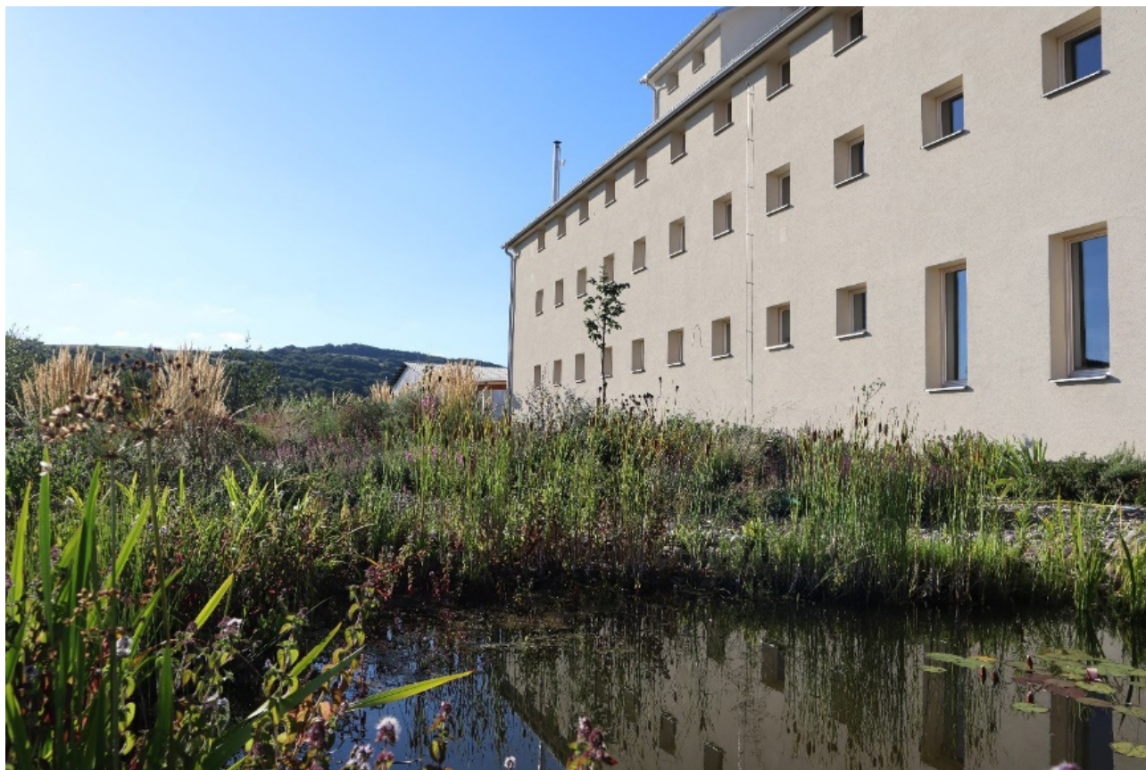
Figure 1 Stormwater retention measures at the reconstructed granary building in ŽiTo v Sýpke, Moravské Lieskové
