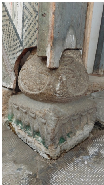
Fig. 16. Romanesque architectural detail.
