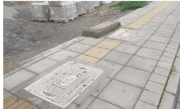
Figure 8-9. Telephone openings and extrusions interrupting the concrete tactile surface (Author, 2025)
