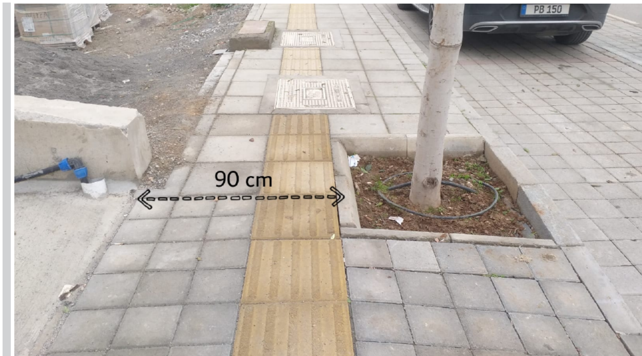
Figure 12. A limited width in the sidewalk to 90cm creates accessibility issues (Author, 2025)
