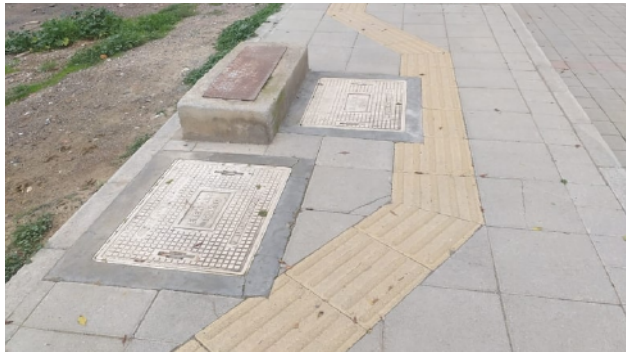
Figure 8-9. Telephone openings and extrusions interrupting the concrete tactile surface (Author, 2025)
