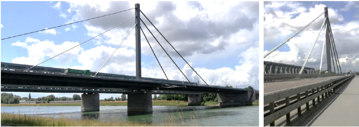
Figure 1. The Rheinbrücke Maxau bridge
