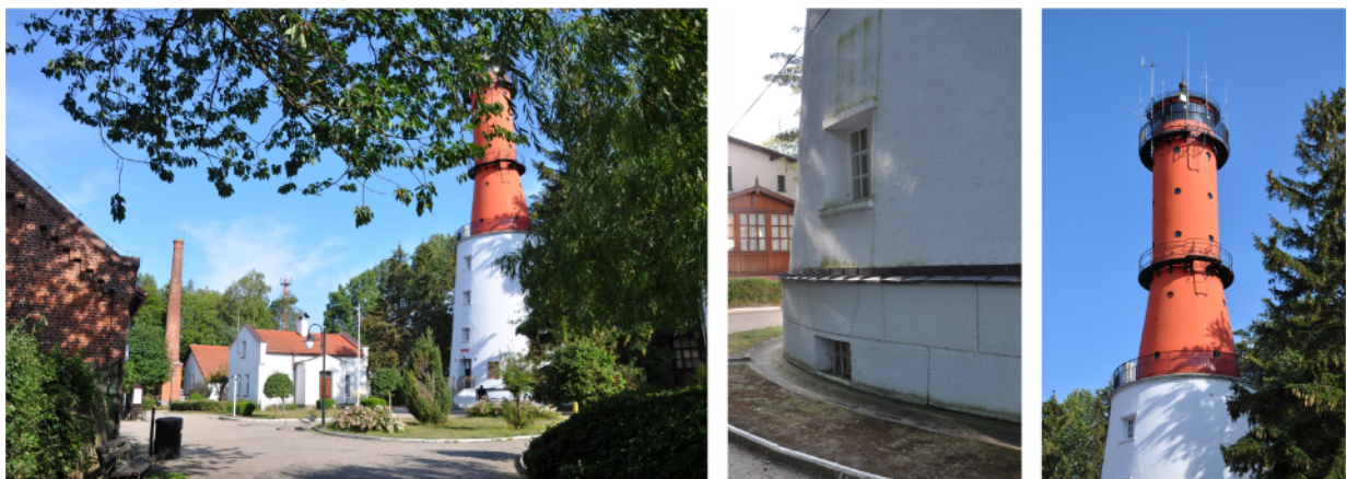
Figure 4. Rozewie I lighthouse. Photographs: A. Pluszczewicz-Fornal
