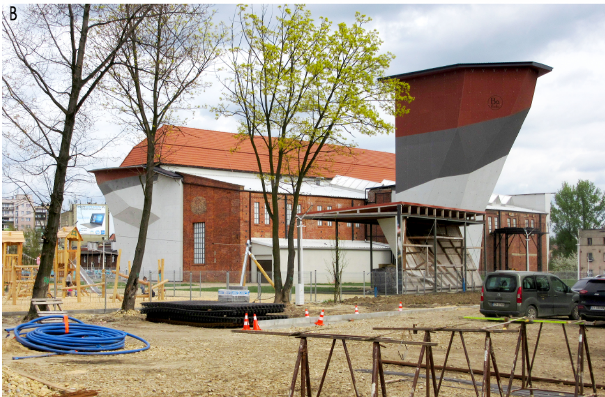
A – construction of the Climbing and Strength Sports Centre (2020)
