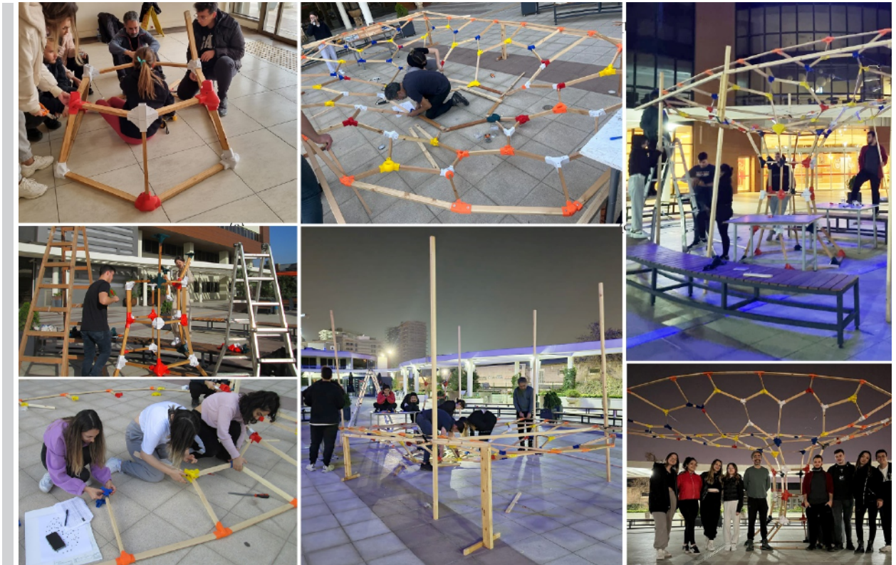
Figure 9. Assembly process of the first prototype in an open area of the campus
