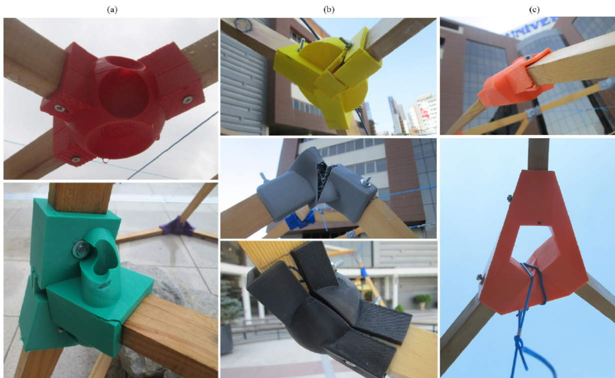
Figure 14. Performance of the nodes during the extreme deformation of the canopy
