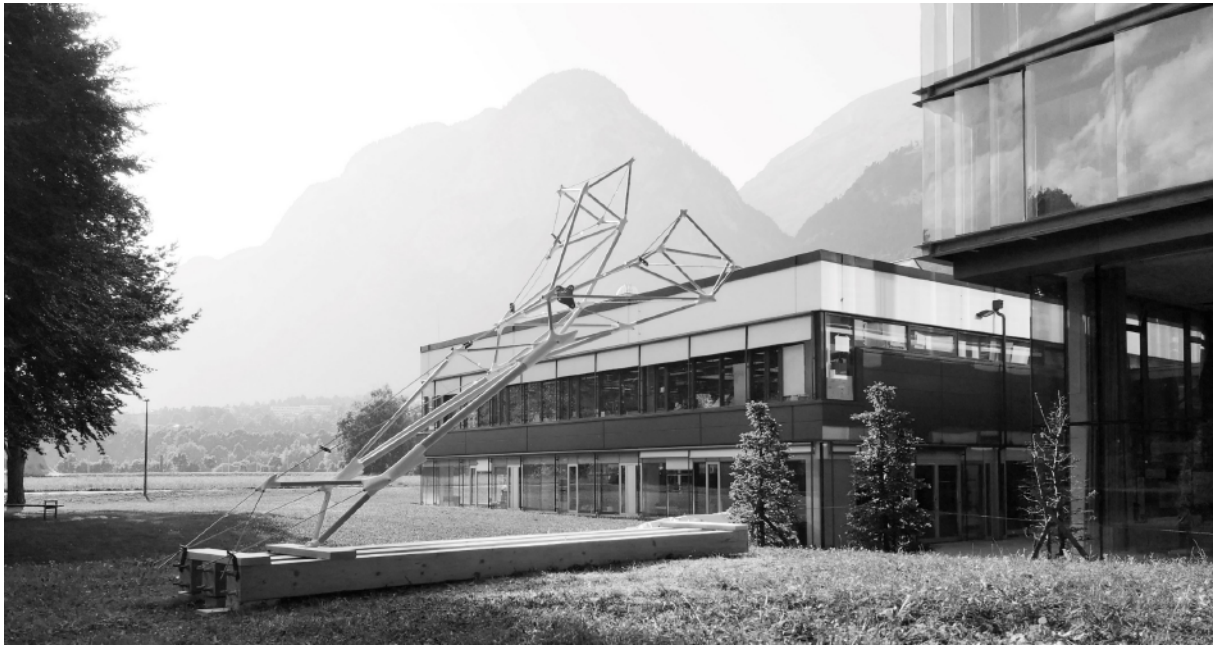
Figure 1. Realized T1 configuration of the Y-shaped, cantilever arm assembled from standardized beech wood profiles and bespoke, 3D printed joints
