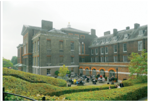
Figure 6. New extension and courtyard to the north of East Front (source: author's archive)
