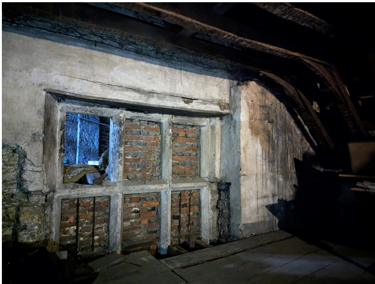
Figure 7. Mullion and transom window of sixteenth-century lodging block. West Sussex, Petworth House, National Trust. Photograph © National Trust Images.
