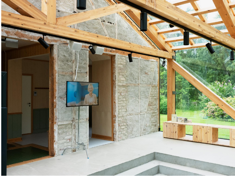
Figure 3. Where Dreams Come Home installed in the glass foyer, 2022. Behind are the remains of the inner timber-framed structure of the original outer wall. Some parts of the floors date from the war years, other are newer. Courtesy of Jakob Ganslmeier.
