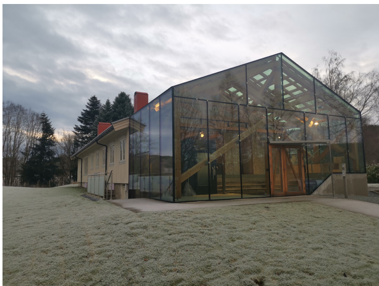
Figure 2. Falstad commandant's house facade, entrance glass foyer, November 2020. Courtesy of: Arne Langås / The Falstad Centre
