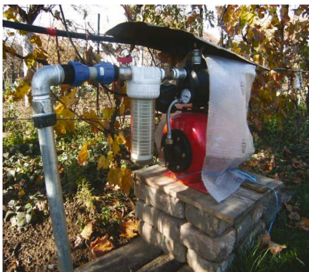
Figure 1. The hydrophore installation
