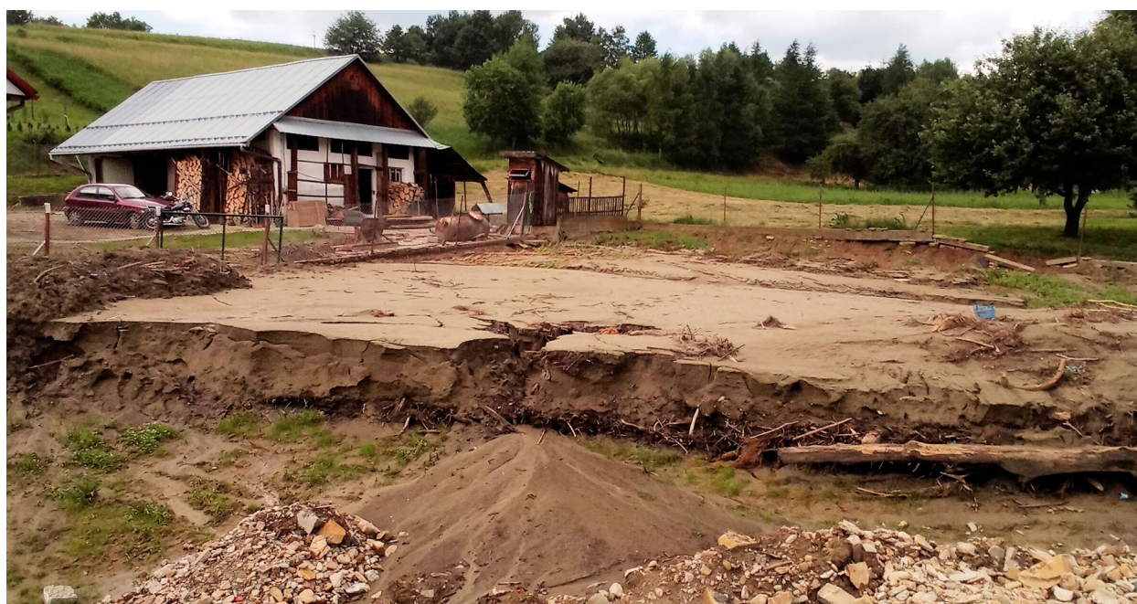
Fig. 9. Delta fan deposits, up to 1 m thick, accumulated in a small valley (a tributary of the Korzonka stream) during the peak of a flood wave backed up by a road embankment and a tree jam blocking the road culvert.
