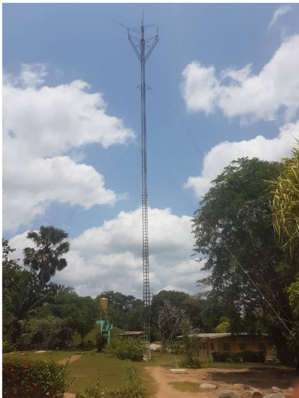
Fig. 4. View of the 50m high tower. Meteorological sensors are installed at the top of the tower, together with the air intake.
