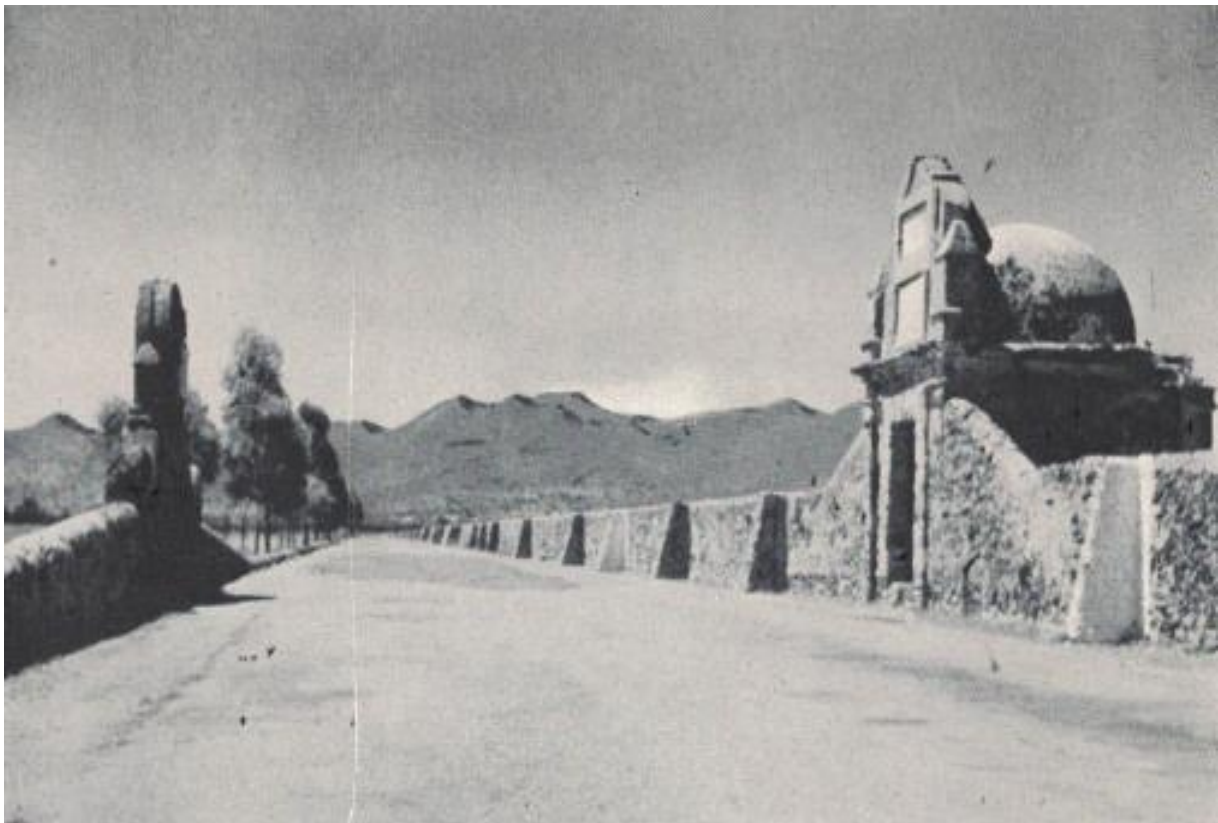
Figure 9. The highway, a few miles outside of Mexico City, circa 1936. Source: Author's personal collection from High Spots of Mexico-Laredo Highway original postcard collection.
