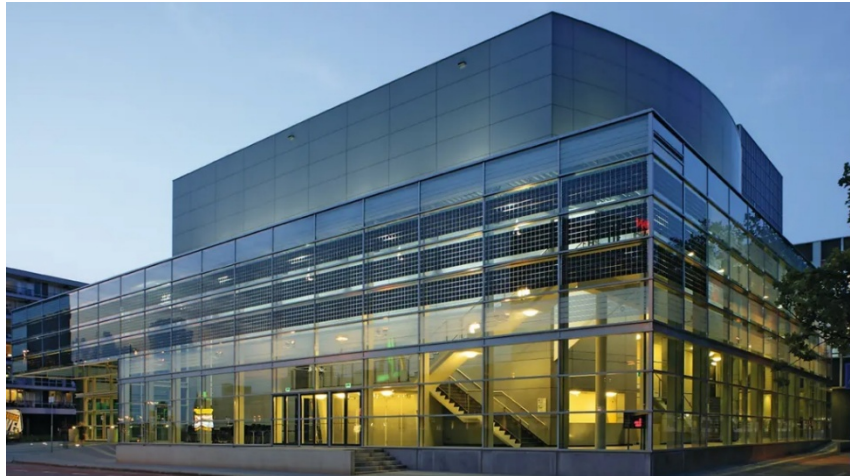
Fig. 1 – Curtain wall facade with photovoltaic panels included (Theatre Heerlen, Heerlen, Netherlands, https://www.schueco.com ).
