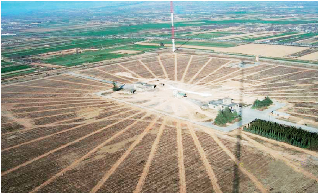
Fig 5.6 the ground counterpoise of the antenna of BPL long wave time service system
