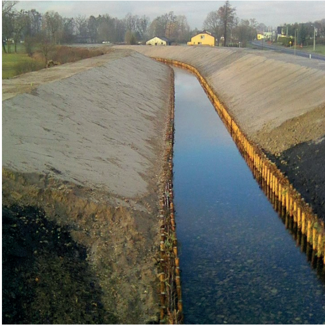
Fig. 8. Topsoiling of slopes
