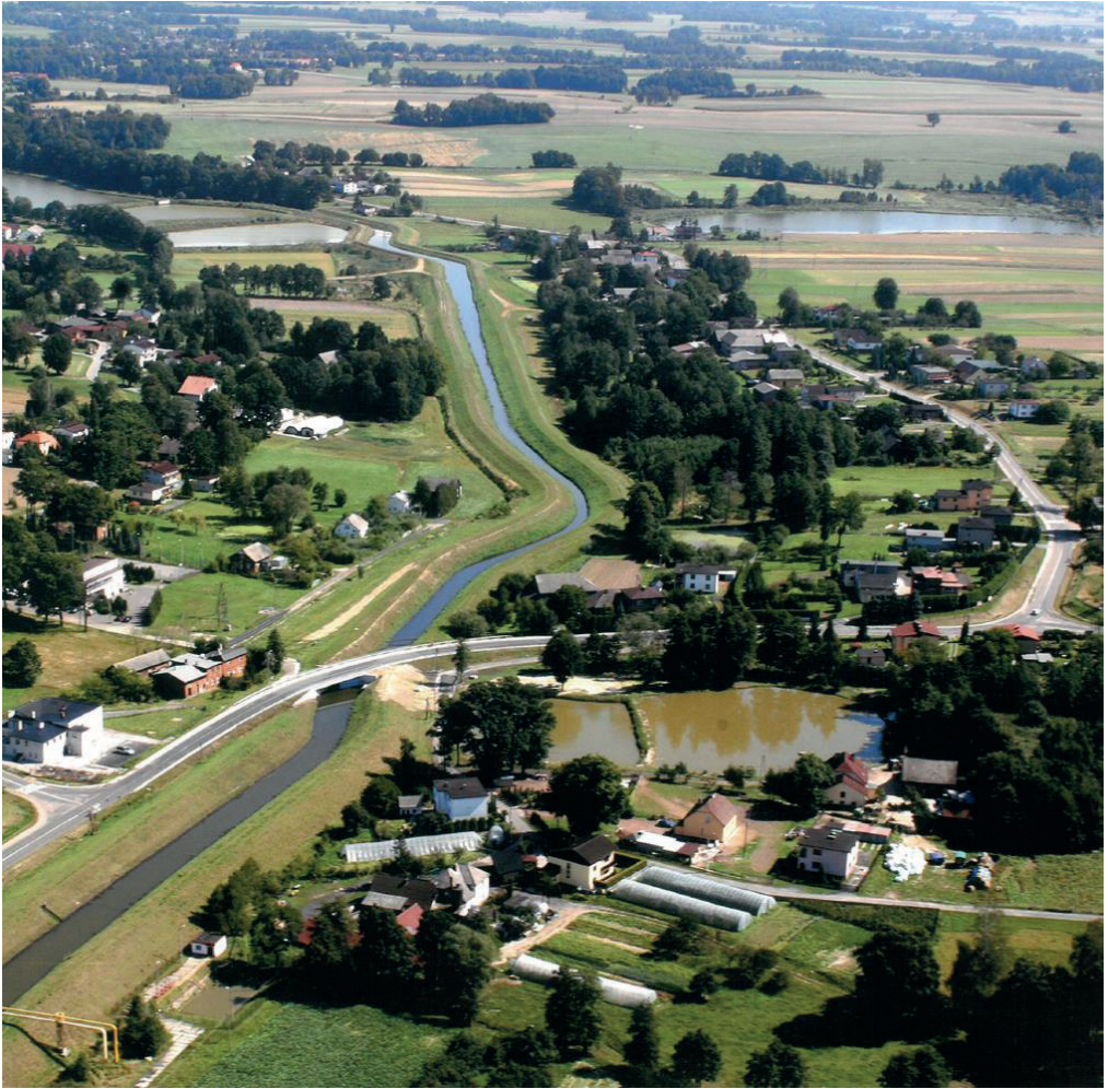
Fig. 10. Completed works after the most recent restoration
