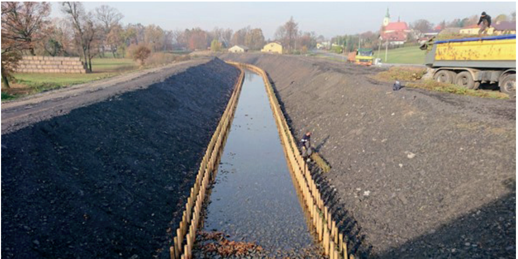
Fig. 9. Fascine construction works
