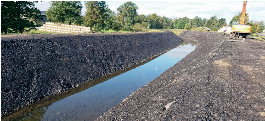
Fig. 7. Preparing riverbed for restoration
