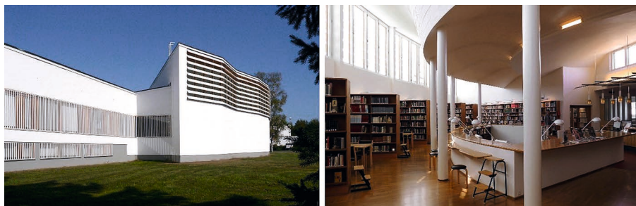
Fig. 7. Seinäjoki Library (1965). A view of the façade with a fan-shaped block with distinctive louvers and a photograph of the interior showing the soft lighting of the reading room space (source: https://www.arkkitehditmustonen.fi/en/projects/aalto-library )
