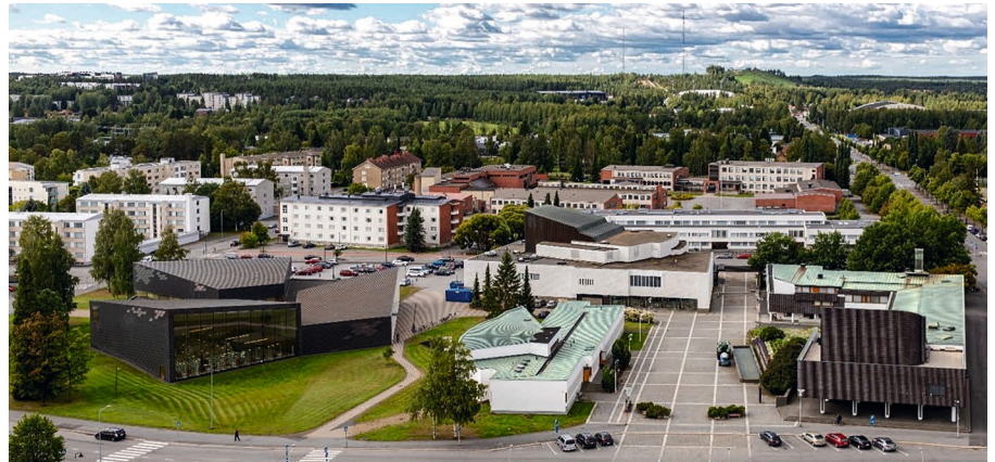
Fig. 5. Seinäjoki Civic Centre. Photo taken after the construction of the new library (photo on the left) with the Aalto-designed buildings: library, town hall (picture on the right) and theatre (in the background) (source: https://www.wikidata.org/wiki/Q4250273 )
