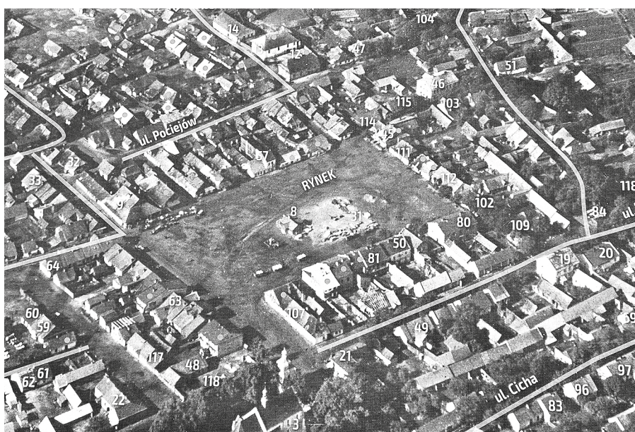
Fig. 9. Aerial photograph of the centre of Zaklików from around 1914 from an exhibition prepared by the Zaklików Town Hall presented in the market square (by D. Kuśnierz-Krupa, 2024)
