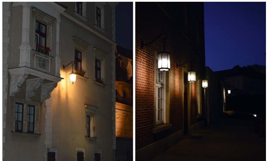
Fig. 4. Façade lamp illuminating improperly (by Jakub Łygan)
