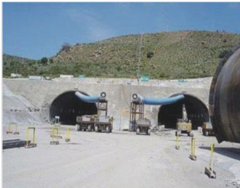
Figure 1: General view of the tunnel T4
