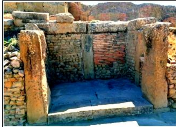
Figure 5: Example of brick usage in the repair of a wall in Timgad (source: Author 2023).
