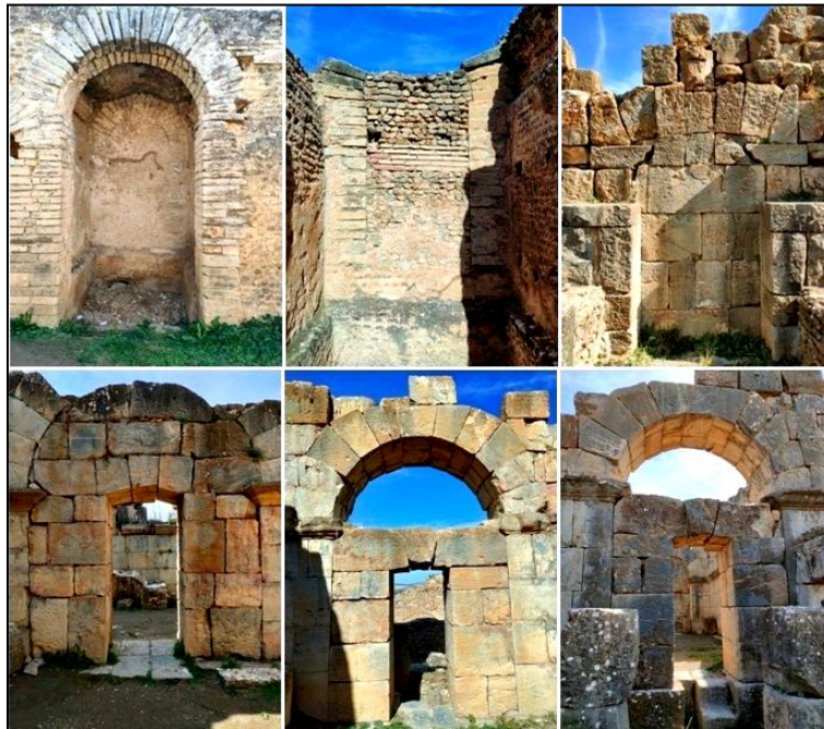
Figure 8: Blocking of openings at Djemila (source: Author 2023).
