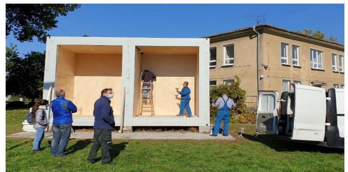
Fig. 3 Process of building two rooms inside the container
