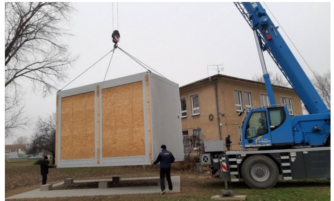
Fig. 2 Process of placing the Twin Rooms container on pre-built concrete foundations
