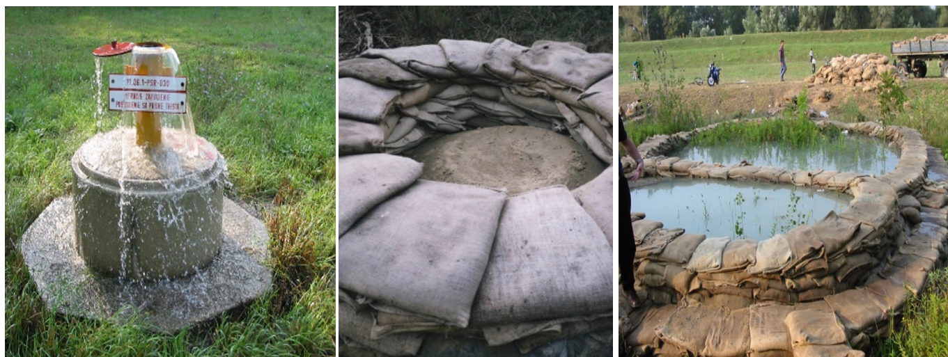
Fig. 1 Accompanying phenomena caused by seepage through the subsoil of the left-side flood control levee of the Danube during flood flows in 2002 (source: Archive of VV Bratislava, TBD Department)
