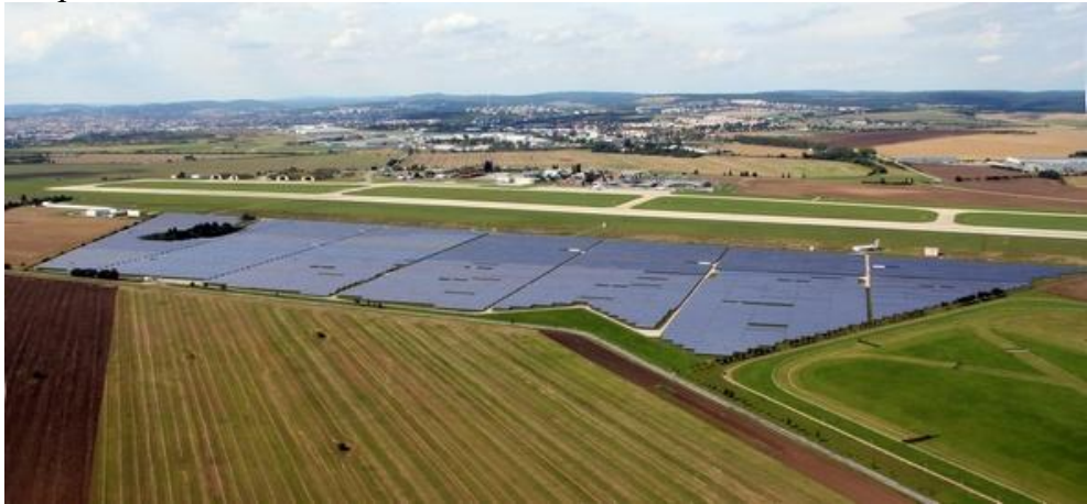
Fig. 1 Photovoltaic Power Plant in Brno (Czech Republic) - Tuřany airport
