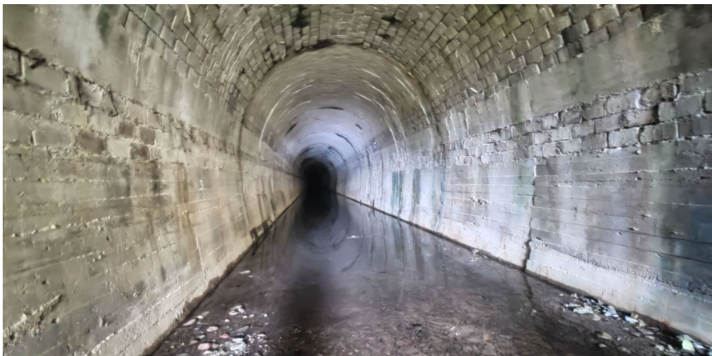
Figure 1. Photo of the tunnel
