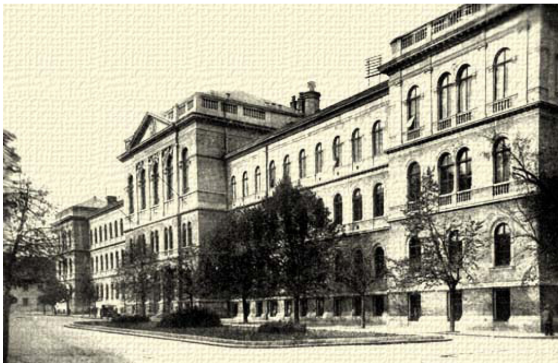
Figure 2. The University of Cluj – Central building on Farkas/Mihai Kogalniceanu Street
