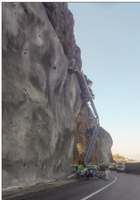
Figure 2. Sprayed concrete at the level of the Cliffs of the Jijel corniche (Photo A. Birouk)
