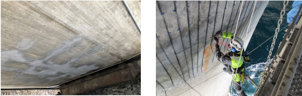
Figure 1 – Left: Spray-applied patch repair of a bridge superstructure. Photo courtesy: Norwegian Public Roads Administration. Right: Installation of anodes for cathodic protection of an offshore oil platform. Photo courtesy: Equinor.
