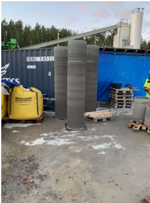
Figure 4 – 3D printed concrete columns in the B.Sc. project during autumn 2021. Photo: T. v. Haslingen.
