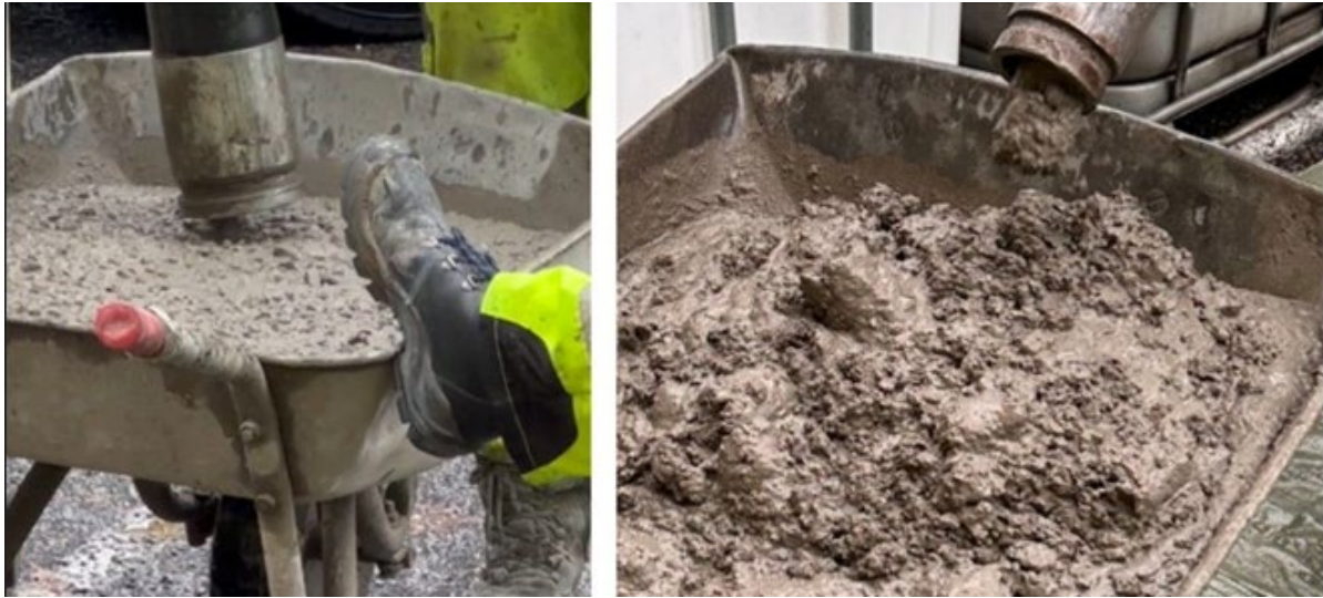
Figure 4 - Left: Fresh concrete after 28-metre boom, homogeneous and no loss of workability. Right: Sudden loss of concrete workability has occurred during pumping.
