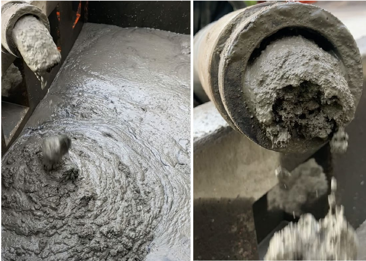
Figure 8 – Left: Concrete experiencing sudden loss of workability with visible separation and inhomogeneous stability. Right: Concrete in the middle of the cross section seems particle dominated, whereas a large amount of matrix flows easily around the particle dominated part.
