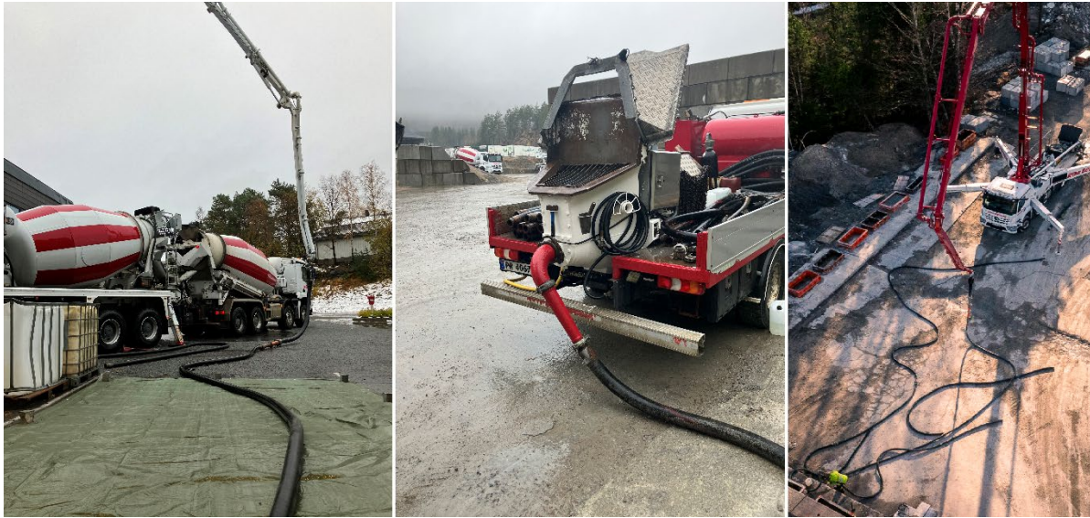
Figure 3 - Left: Setup of pumping with pump mixer and 10 m extension hose following the boom. Middle: Setup of line pump: concrete hopper, U-bend, reducer, and extension hose. Right: Setup of pumping with 43 m boom and up to 30 m extension hoses.
