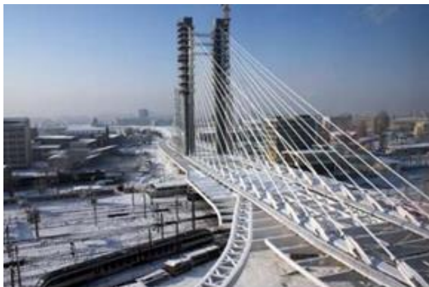
Fig.2. Basarab Passage - drawbridge (suspended)
