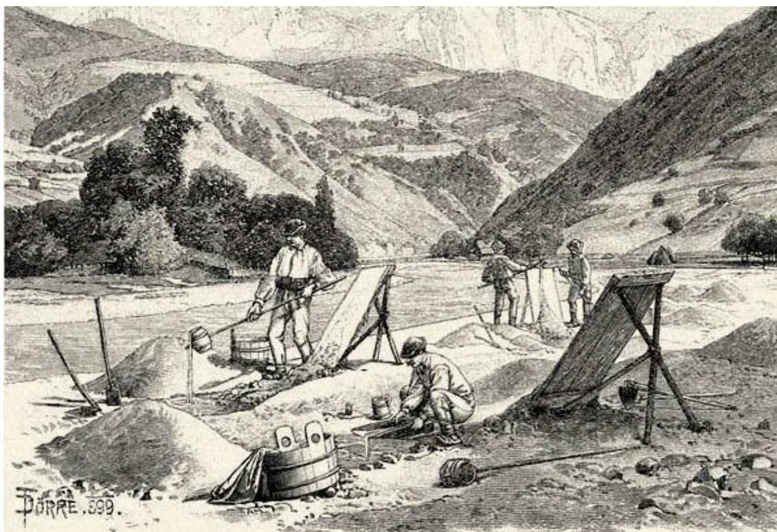
Fig.5. Mining of alluvial gold [7, page 113]
