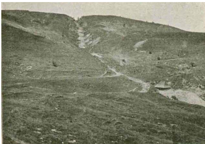
Fig.6. The hushing dug by the Romans on the southern slope of Corabia
