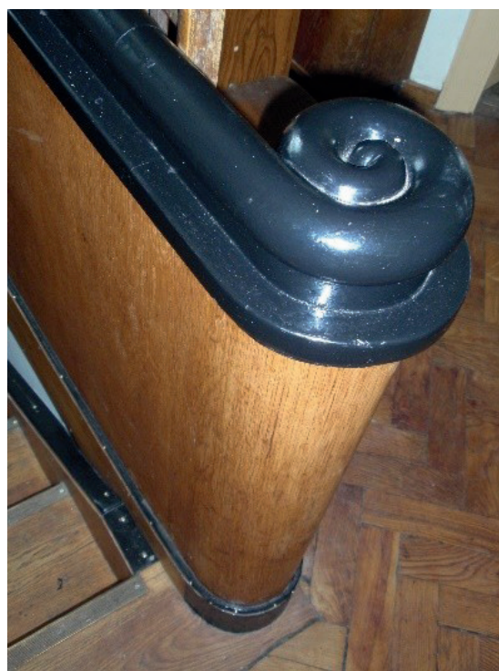
Fig. 10a. Decorative wooden finish of the stair railing in the house of Jablonskytė-Petkevičienė, designed in 1930s by arch. Landsbergis-Žemkalnis. In the interior, the dominant colour of natural oak is combined with black details: furniture plinths, cornices and handles, painted baseboards, stair railings. Photo by Preišegalavičienė, 2010
