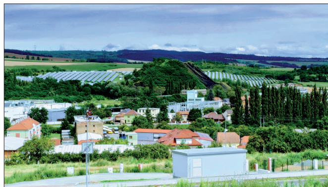
Fig. 6: PV power plant constructed on a former coal ash dump in the town of Oslavany. The landscape is dominated by the heap of boiler slag from an already demolished coal-fired power plant (the slag is gradually processed as an ingredient in building materials) Photo: B. Frantál
