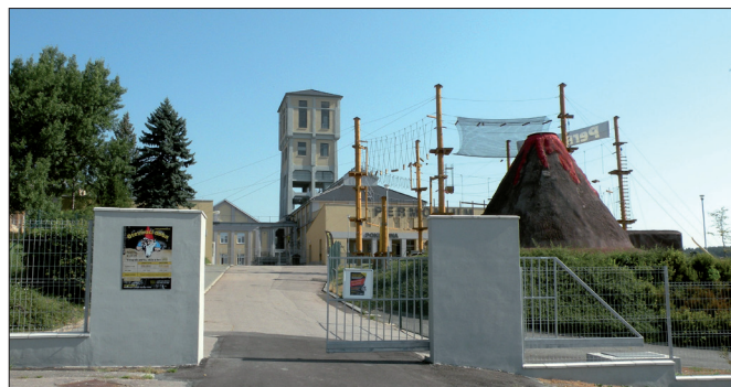
Fig. 11: Permonium Park – former complex of the Kukla mine in Oslavany town recycled into amusement park Photo: B. Frantál
