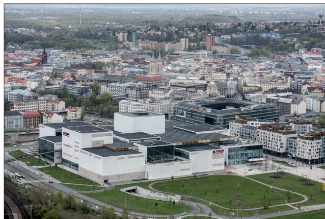
Fig. 8: Forum New Karolina – the shopping mall, residential houses and office spaces constructed after demolition of a former coal industrial complex
