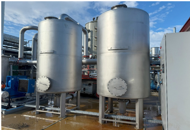
Fig. 7. Activated carbon filter.
