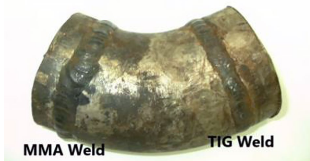
Fig. 5. Failed elbow showing poor welding at one side (left) weld joint
