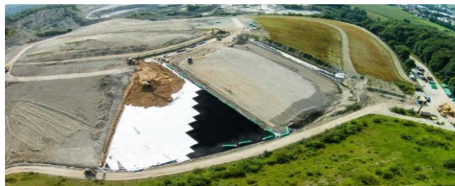
Figure 3. Landfill under construction or expansion covered by a white membrane, which is a waterproofing layer, essential to prevent the infiltration of toxic substances into the soil and groundwater
