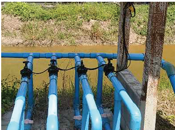
Figure 3: The demonstration of the installation pump system and solenoid valves.
