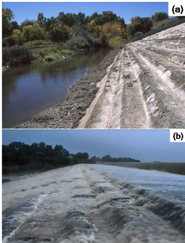
Fig. 1. (a) The auxiliary stepped spillway of the Leyden Dam in Colorado, USA; and (b) overtopping flow along the chute during a storm event (after Hansen and Fitzgerald 2016)
