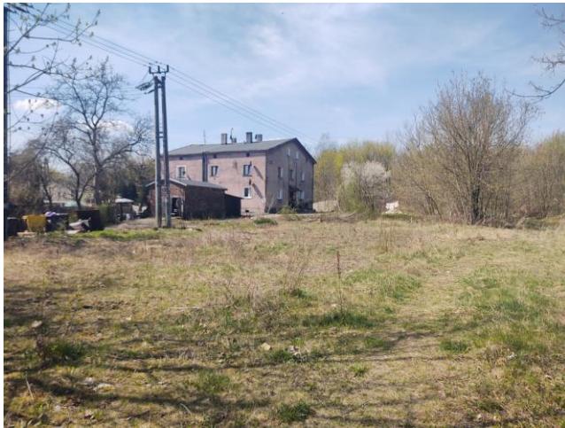
Fig. 2. Former water-shaft at "Jacek" mine, now residential house (Sosnowiec-Bobrek) (Source: author)
