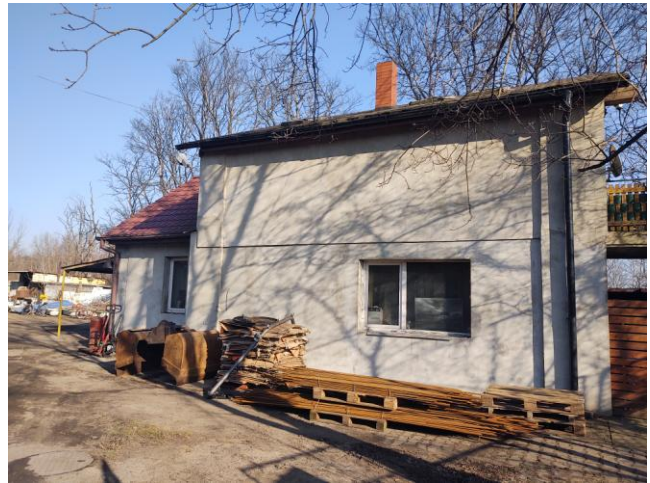
Fig. 3. Administrative building and area of the former "Barbara" shallow coal mine in Sosnowiec (Source: author)
